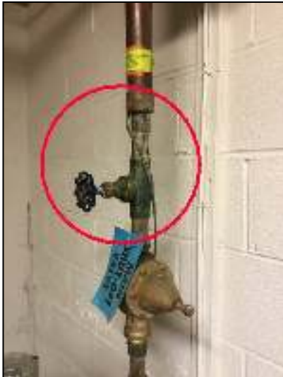
Repair leaking valve at main water line. Seal wall penetration.
