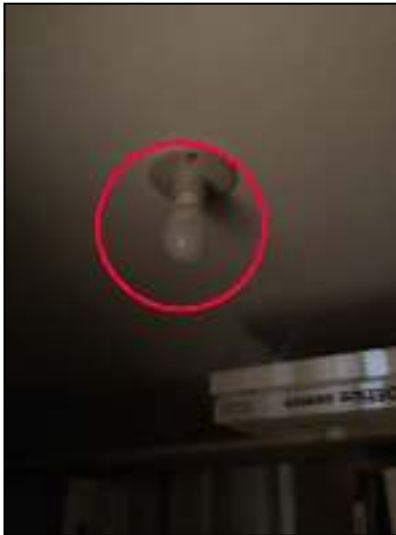
Install globe on basement storage room closet bulb
