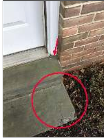
Repair stone steps at back left garage door.
