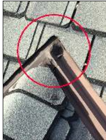
Properly seal all top metal flashing on roof terminations.
