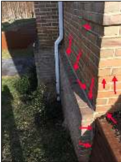
Repair brick joints at left end lower level front left corner.
