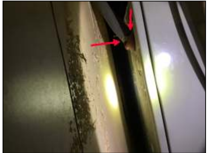
Install proper electrical connector on furnace in basement. Left side.
